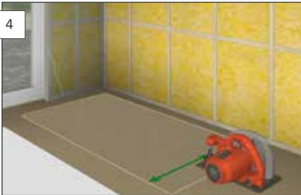
Measure and cut the first panel (panel width must be minimum 450 mm). Be careful with the panel's profile.
