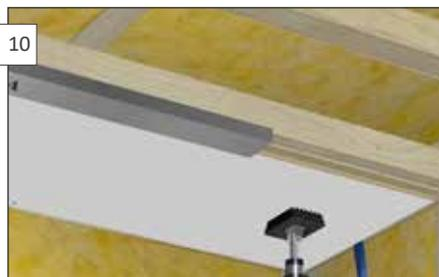
To fit the last panel, use a crowbar to close the profile. Use the guide rail for a final adjustment.
