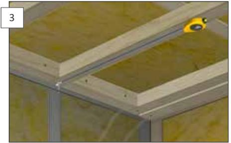
Install the first row of panels following the line. Remember that there must be a 10-mm clearance by all fixed structures. It is essential that the underlay is perfectly straight. Any unevenness in the framework **MUST** be corrected before installation.
