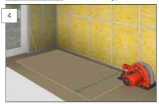
Measure and cut the first panel (panel width must be minimum 550 mm). Be careful with the panel's profile. When using a saw, place the panel with the foil facing down
