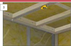
Install the first row of panels following the line. Remember that there must be a 10-mm clearance by all fixed structures. It is essential that the underlay is perfectly straight. Any unevenness in the framework MUST be corrected before installation.
